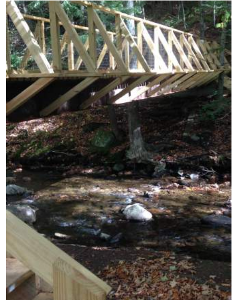
(Above) The new bridge across Mill Brook, built in 2016 with special attention to protecting the brook and providing access for many types of use in the Town Forest...
